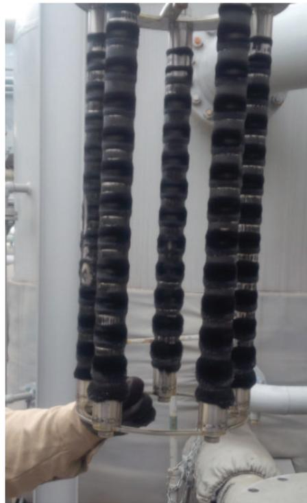
Figure 4. Black Powder contamination captured by the magnetic elements.
