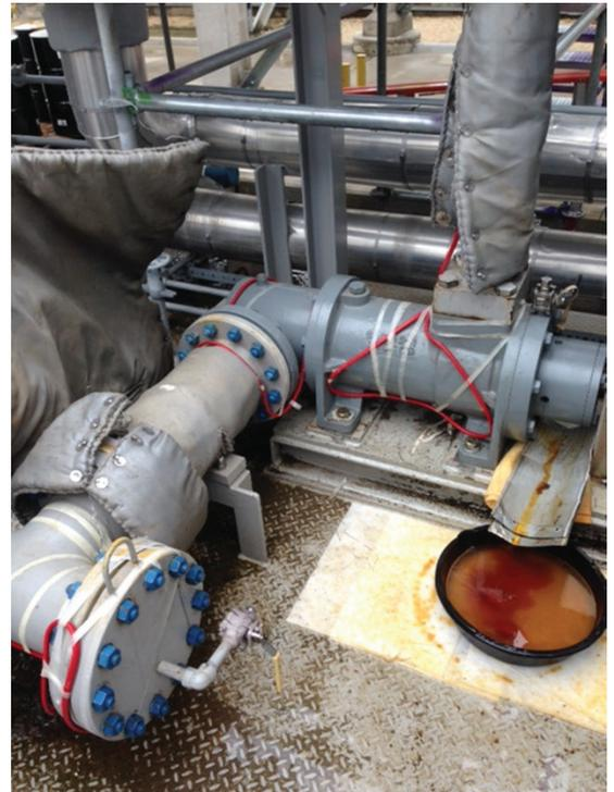
Figure 1. Constant seal leakage from IMO Lube Oil Pumps.
