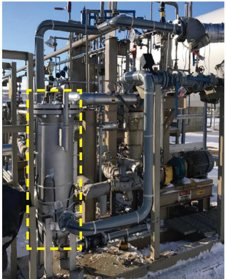
Figure 1. The installed BPS Magnetic Separator
