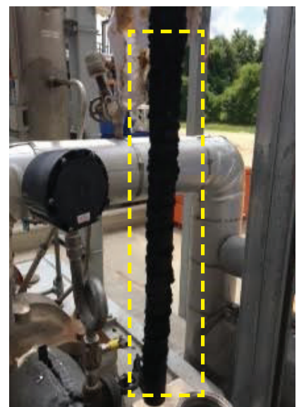
Figure 2. Black Powder collected on the Magnetic Separator element
