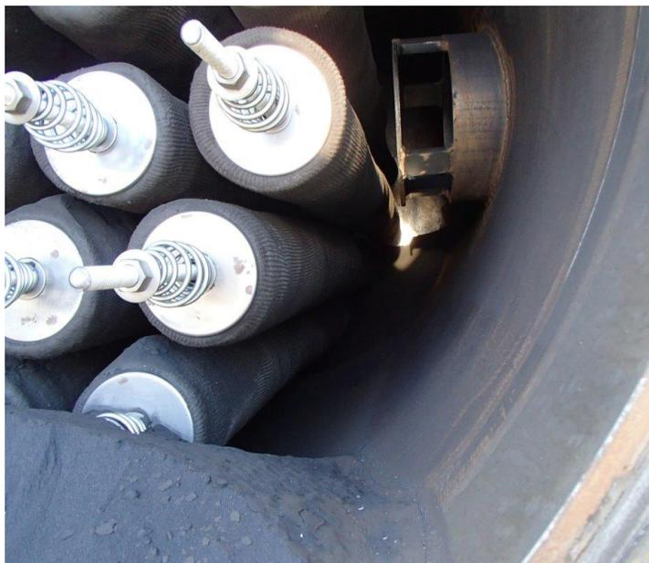
Figure 1. Contamination not captured by conventional filters.
