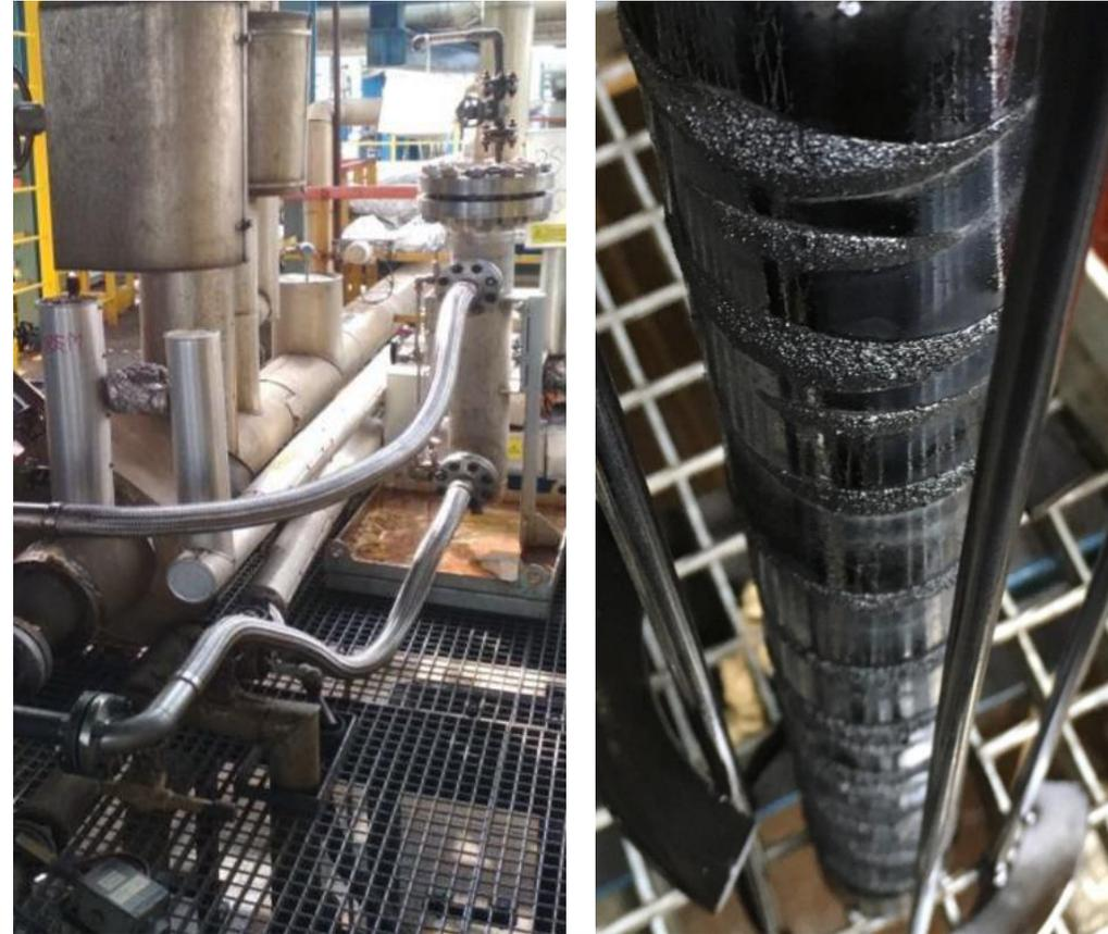
BPS magnetic separator installed in the HDS amine system during testing, as well as contamination captured on the magnetic separator element.
