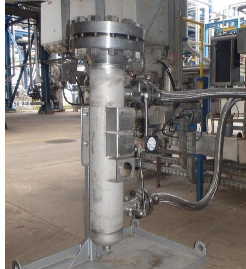
BPS magnetic separator installed in the hydrocracker fuel gas system.
