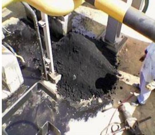
**Fig. 1.** Black powder accumulation on metering station.
